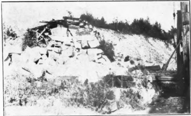
End of Inclined Tracks from Top of Quarry to Crushing Plant. Stone is removed by derrick at right
